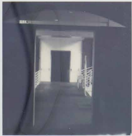
1 I'm looking at the foyer I'm looking at the doors open
